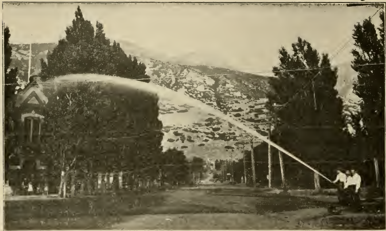
Street Scene in Farmington—Notice Water Pressure From City Mains.
